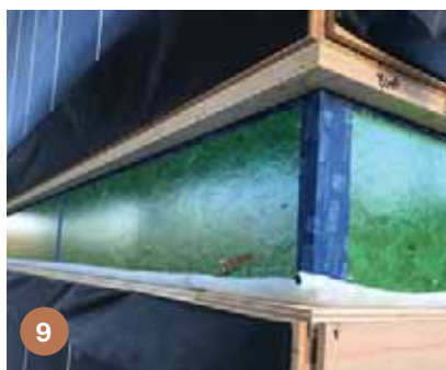
1 Insulated foundations with services for heat pump and ventilation unit in small plant room on ground floor (avoiding ducting in attic); 2 Thermally broken double soleplate overlapping upstand of insulated raft foundation to eliminate thermal bridging at wall to floor junction; 3 Thermal bridge-free door thresholds formed with Bosig Phonotherm structural insulation board, sealed with Extoseal Encors waterproof sealing tape; 4 Metsa Wood FJI engineered timber I-studs minimise repeat thermal bridges through walls, while Medite Vent breathable racking board ensures the wall is water vapour diffusion open to the outside; 5 Metsa Wood Kerto LVL used to form strong L-corners to allow insulation to fill into corners to eliminate thermal bridging. Also used for top and bottom rails; 6 Gutex Therminstal fitted around window and door reveals to eliminate thermal bridging; 7 3 mm expansion gap between Smartply Airtight OSB panel edges, prior to joints being taped with airtight tape; 8 Closed panel to soleplate junction. The Smartply Airtight OSB and Medite Vent breathable panels oversail the soleplate for a precision fit and to facilitate mechanical fixings through the panels into the soleplates; 9 Bespoke airtight intermediate floor junction using Smartply Airtight. Floor is set back and insulated with rigid Gutex Multitherm wood fibre insulation to eliminate thermal bridging at the floor perimeter; 10 Intermediate floor of Smartply Strong Deck (OSB/4) T&G, screwed to Metsa Wood FFI-Joists, for superior strength and acoustic performance.
